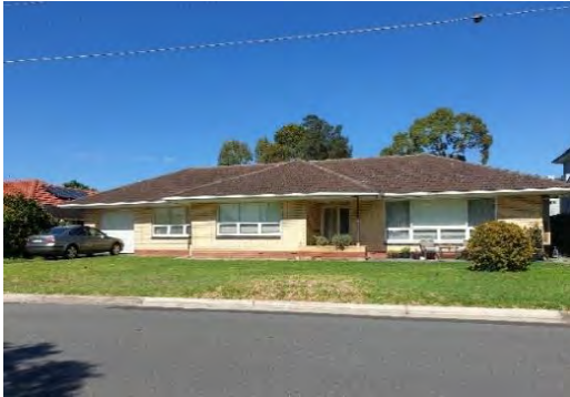
C5 Image 2: 13 Old Drive is an example of a 1960s dwelling which is typical to this area, which has undergone little alteration.
