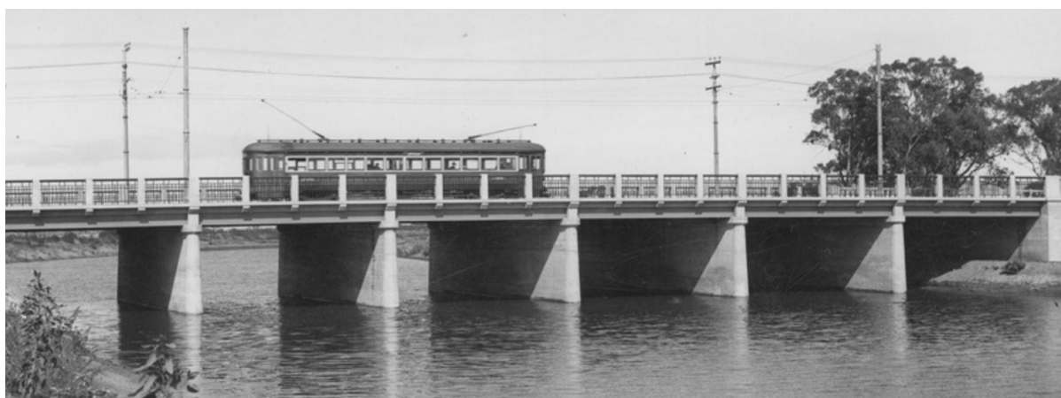
Figure 22 c.1930s photograph of Kidman Bridge at Henley Beach Road, Lockleys (SLSA B 9815)
