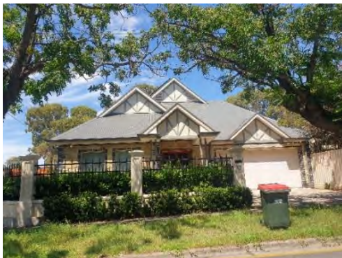
C4 Image 5: 12 Malurus Ave is a recent dwelling which (while not perfect) has been designed to complement the character of the area and "fit in".
