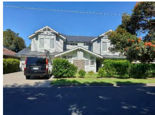
C5 Image 6: 15 Old Drive is a contemporary dwelling which is incongruous with the area, mostly due to its height, roof form and materials.
