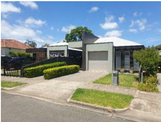
C3 Image 3: 42 and 42A Albion Ave are example of mid-2010s dwellings which has features in conflict with the character statement (prominent garage, fenestration proportions, roof form, modern portico, limited setbacks).
