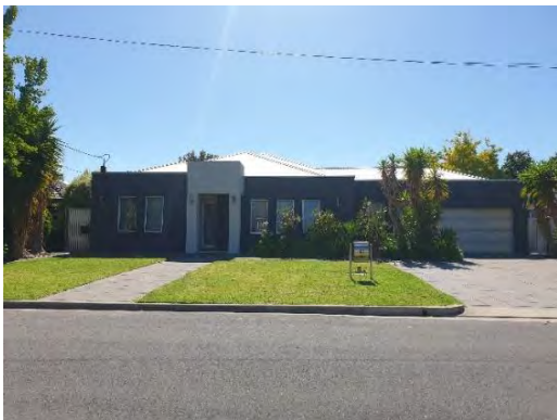
C5 Image 5: 13 Sycamore Ave is a contemporary dwelling with complementary proportions but with other features which are not as complementary.
