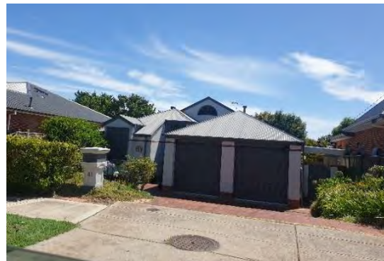
C4 Image 6: 41 Malurus Ave is a recent dwelling which displays few features which complement the character of the area (dwelling proportions, prominent garage, roof form).
