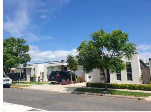
C6 Image 2: Dwellings at 39 Kintore which are contemporary dwellings located within the CAO but are not complementary to the character of the area.
