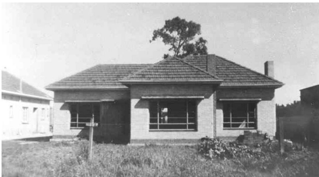
Figure 28 Construction of a home in Daly Street, Kurralta Park, c.1955 (West Torrens Historical Society, LH0499)
