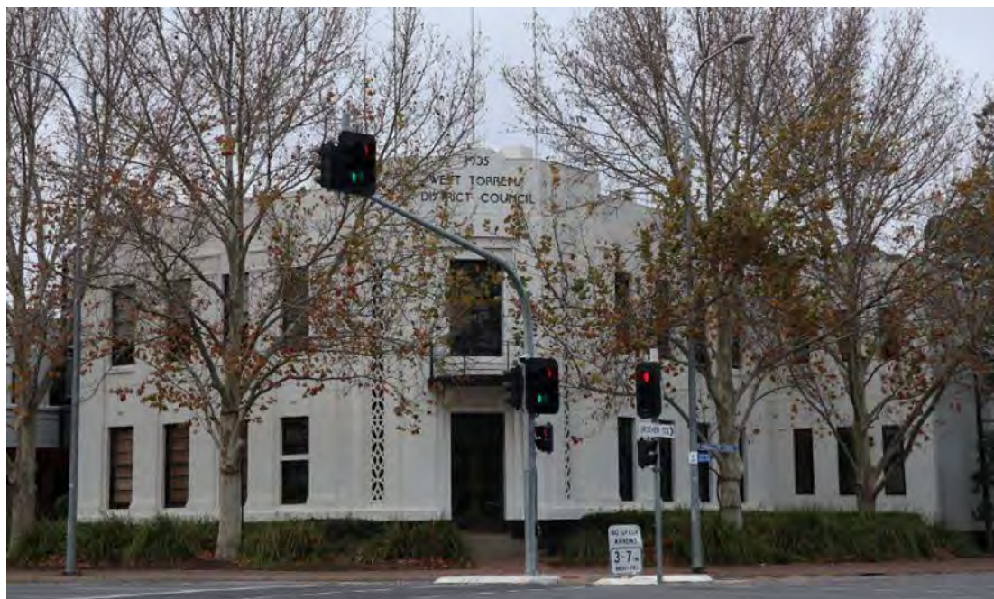
Figure 25 West Torrens Council Chambers, Sir Donald Bradman Drive, Hilton ( https://www.flickr.com/photos/31967465@N04/52265936353 , accessed 22/12/2023)
