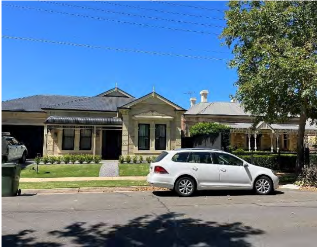
Figure 35: Reproduction dwelling at left; original / early dwelling to right – note garage under main roof at left.
